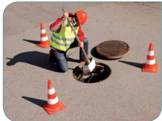
Pic: Installation of SQ in the sewer
